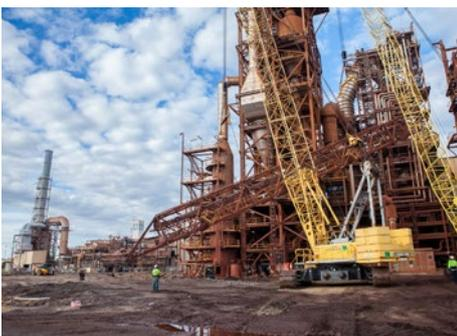
The salvaged items included the 65 metre high, 1200 tonne Coal drying and grinding structure, the Flue Gas Desulphurisation plant, Hot Metal Handling equipment including an 80t induction furnace, the Hot Metal Desulphurisation plant, Off Gas Scrubbing and Cooling infrastructure, and a 25 megawatt power station. Carrying out lifts of up to 108 tonne, the dismantling process relied heavily on complex engineering lifts using large crawler and mobile cranes.
